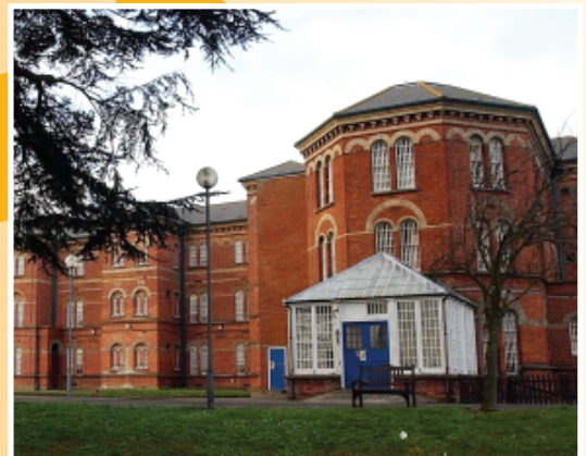
Over the past 12 years, 4C has worked with the Trust on many projects, including a voice and data infrastructure replacement at Broadmoor Secure Hospital
